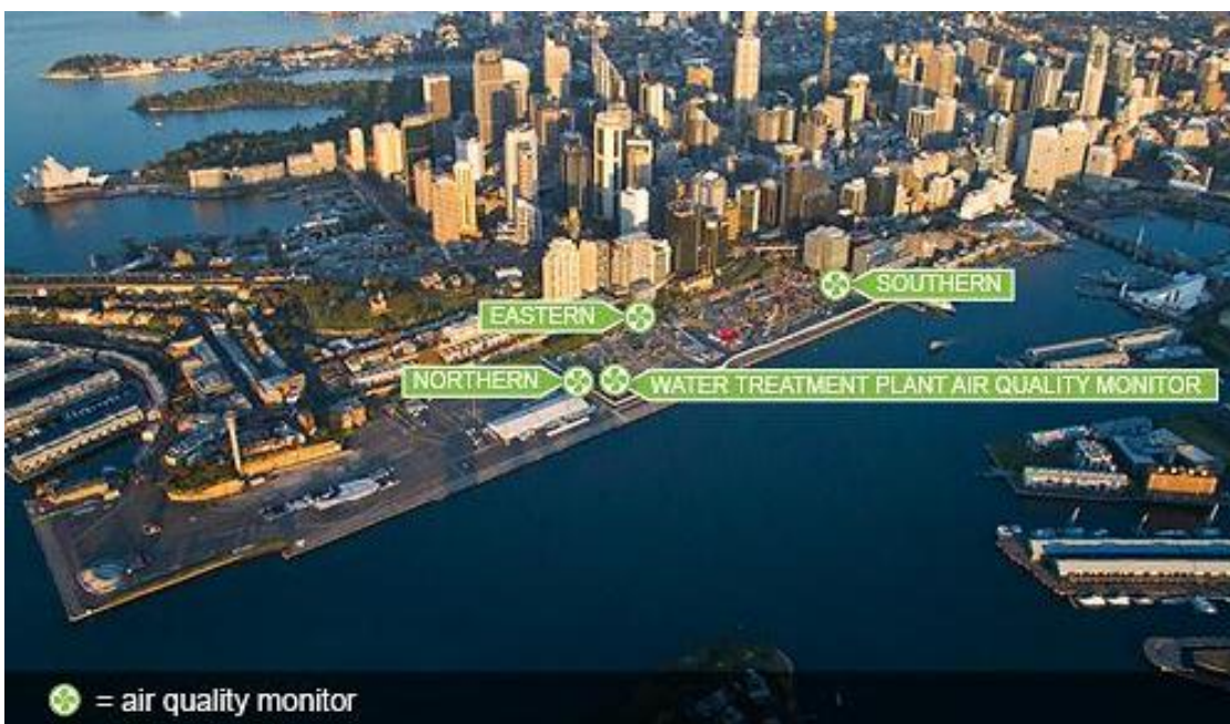
Approximate locations of air monitoring equipment
