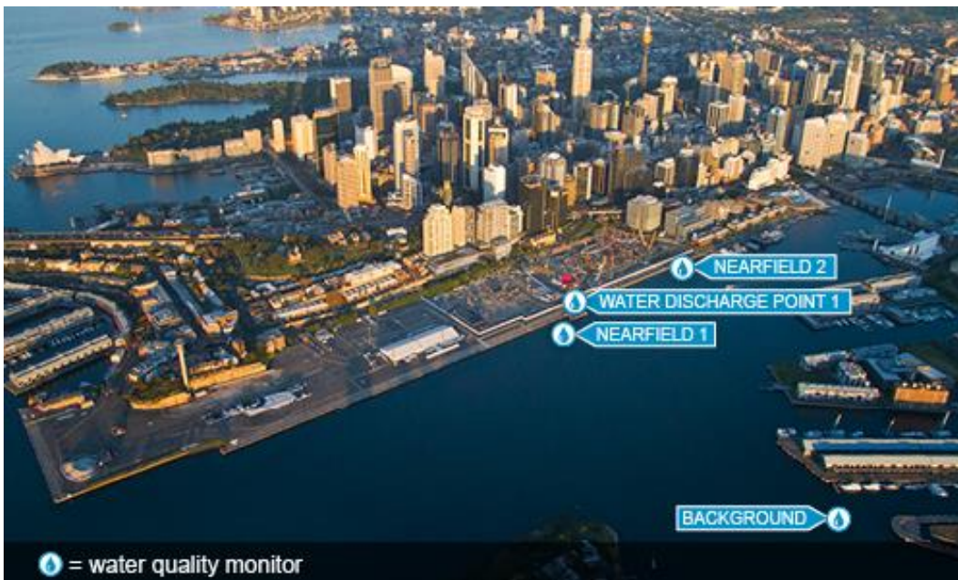
Approximate locations of water monitoring equipment
