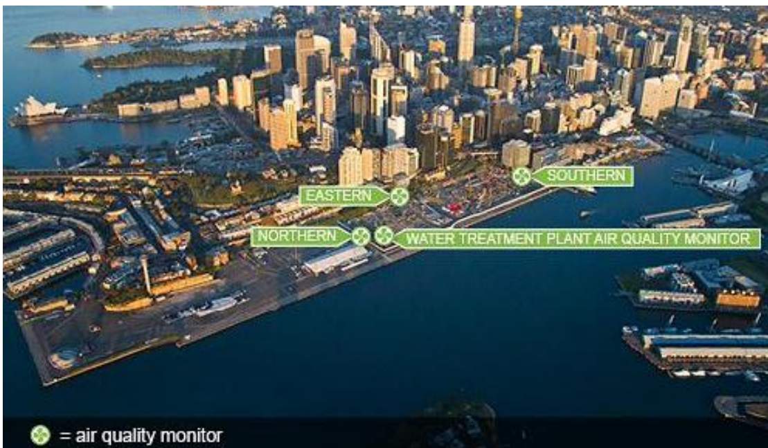
Approximate locations of air monitoring equipment
