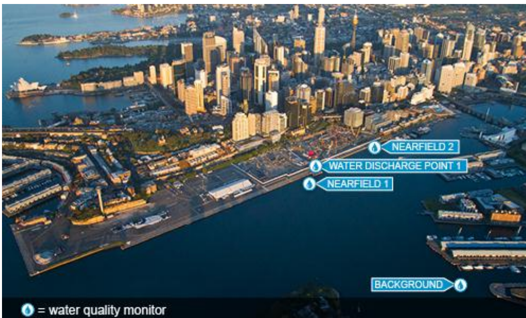
Approximate locations of water monitoring equipment
