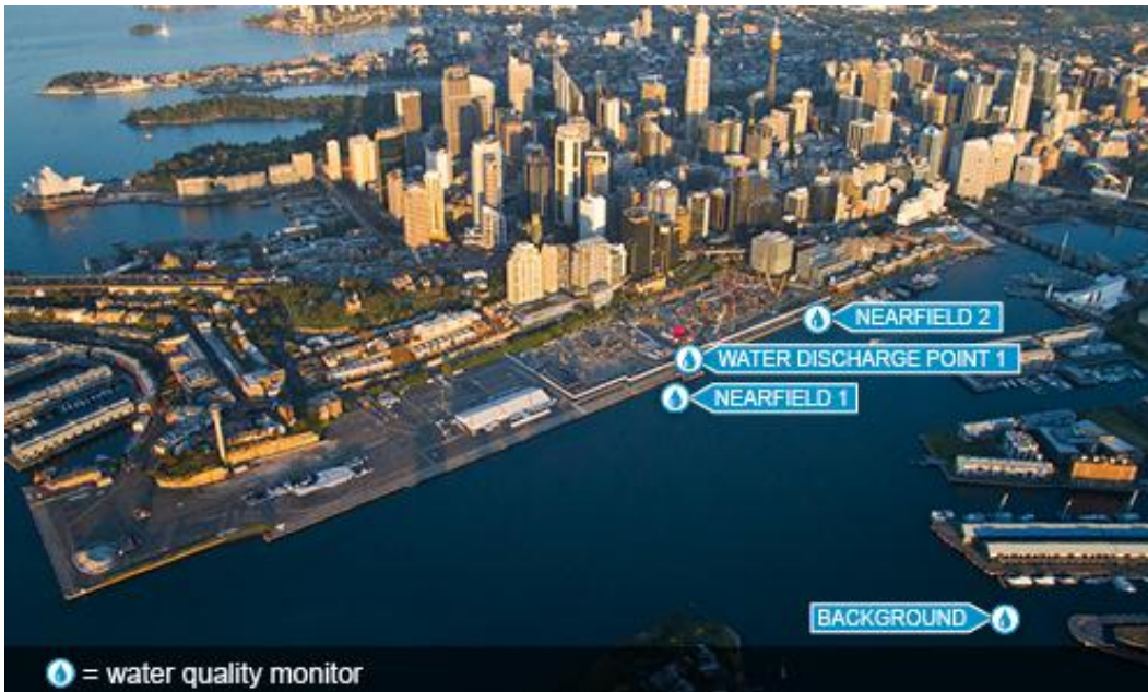
Approximate locations of water monitoring equipment
