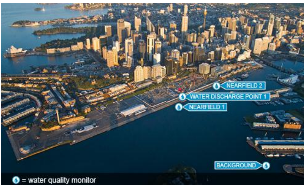
Approximate locations of water monitoring equipment
