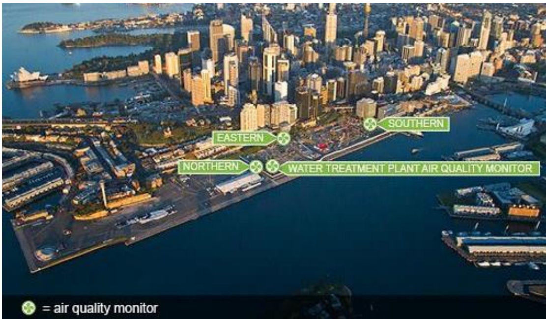
Approximate locations of air monitoring equipment
